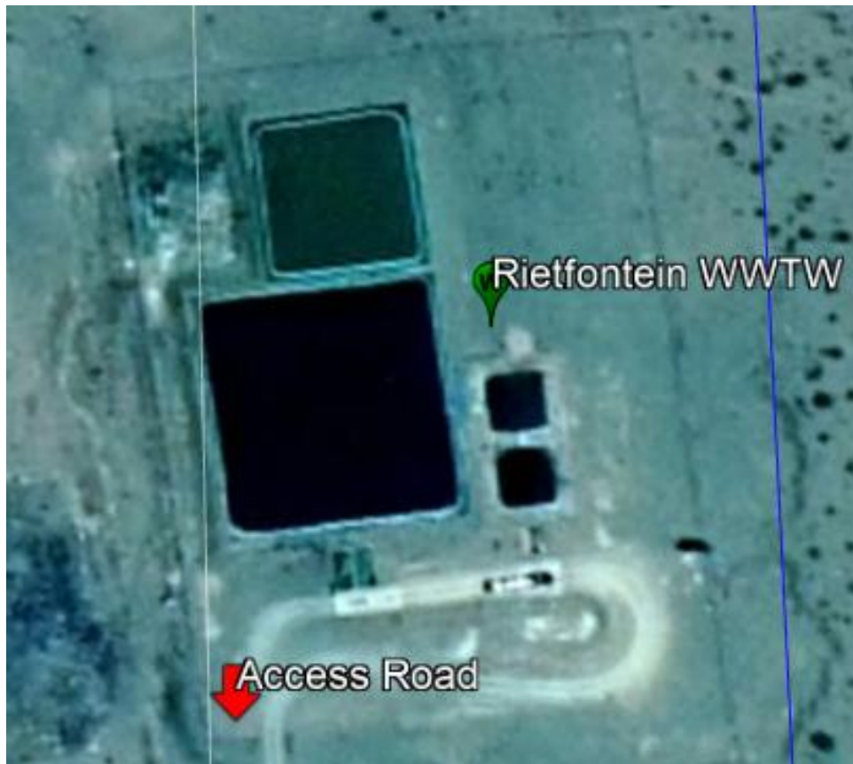
Figure 1 - Existing WWTW oxidation ponds to be refurbished and upgraded.
